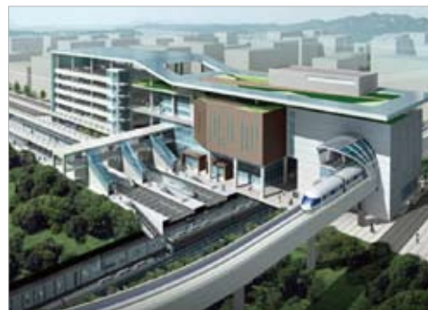
Figure 7.12. Aerial view of the multimodal transit center
