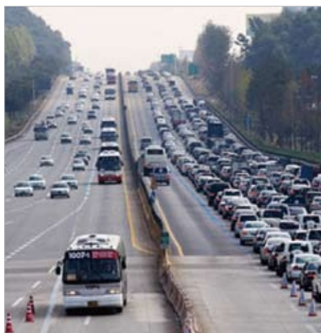
Figure 7.6. Exclusive bus lanes on the Gyeongbu Expressway
