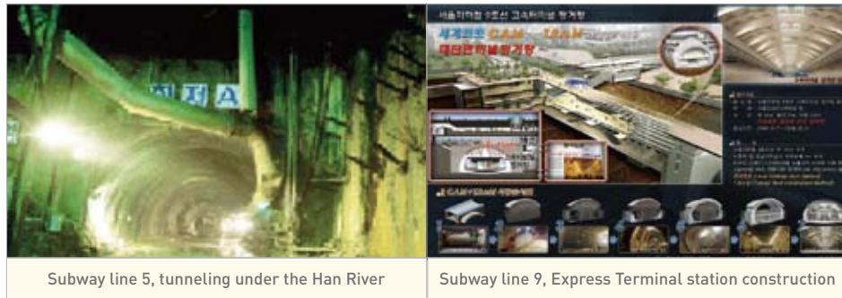
Figure 8.15. Seoul subway construction process
